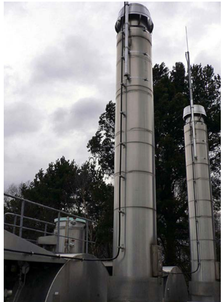
Installation of HVI®Conductors in a hazardous area.
