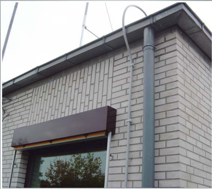
DEHNconductor system HVI® conductor
