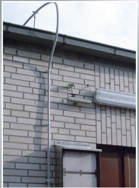
DEHNconductor system HVI® conductor
