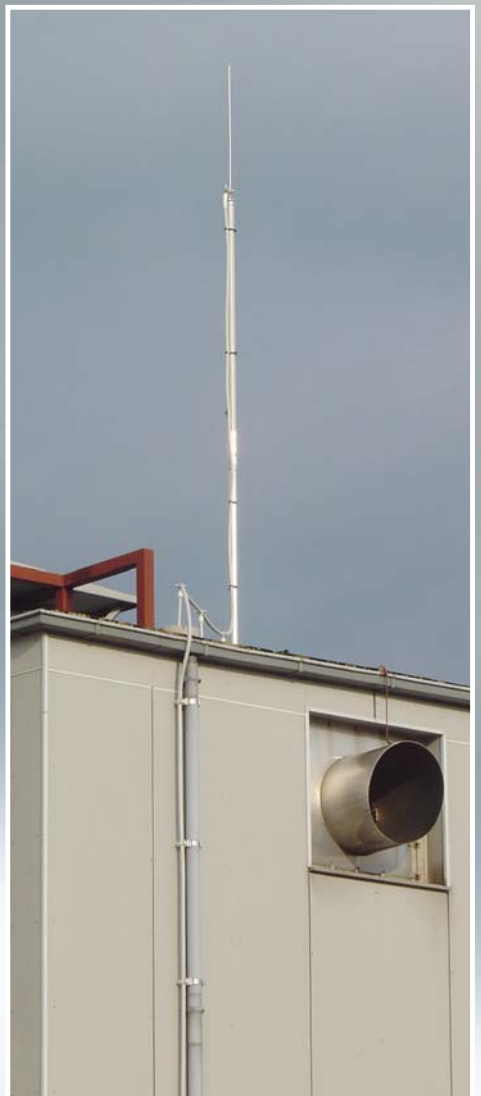
DEHNconductor system HVI® conductor
