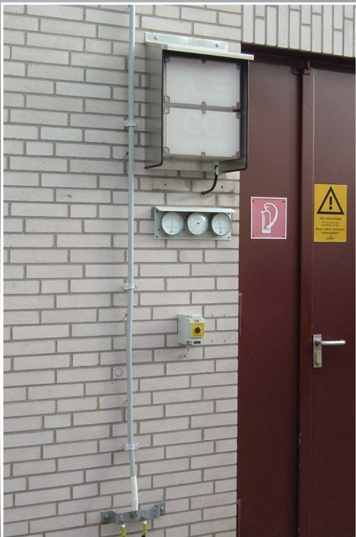
DEHNconductor system HVI® conductor
