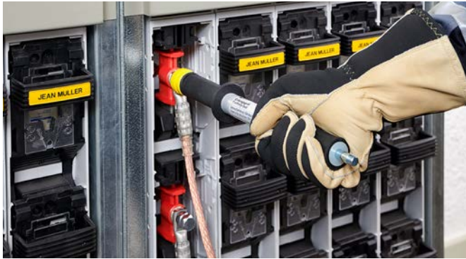
Attaching a partly insulated earthing and short-circuiting device using an earthing handle of type TI.
