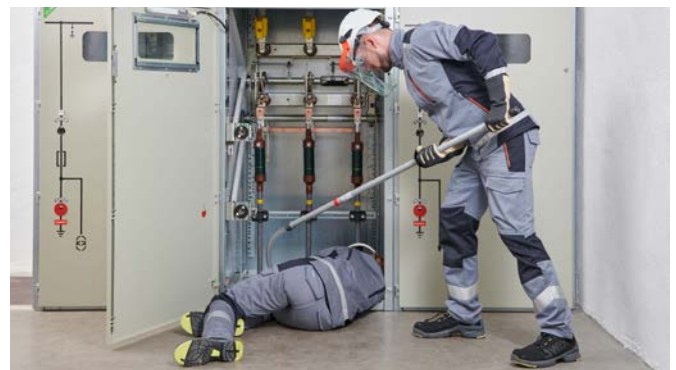
Insulated RST rescue rod used to rescue a victim of electrical shock from the live working zone.
