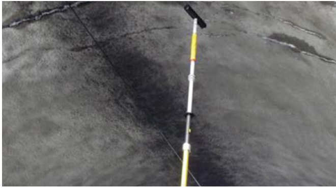
Removing icicles on a tunnel entrance.
