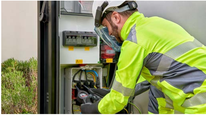
Fitter wearing protective equipment for charging post maintenance.
