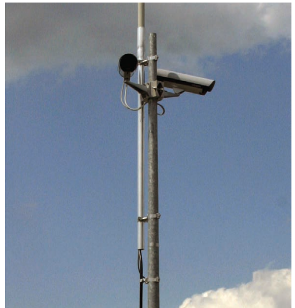
Figure 9.22.4 HVI Conductor installed at a pylon
