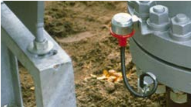
ATEX and IECEx-certified isolating spark gap for lightning equipotential bonding according to IEC 62305 with flexible cable connection.
