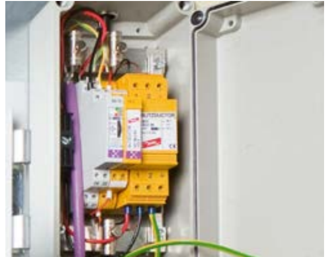
Compact DIN rail mounted surge protective device with screw terminals for multi-core lines.
