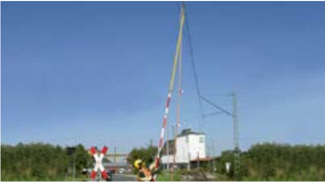
Attaching a railway earthing device.
