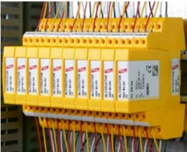
Pluggable and universal multipole surge arrester for use in information technology systems.
