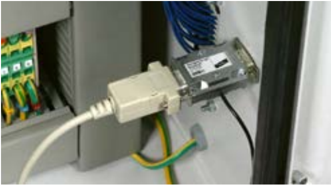
Surge arrester with D-SUB connection (pin / socket version).
