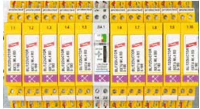
Installed DEHNrecord condition monitoring system
