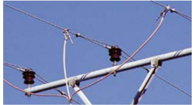
Phase screw clamps used on an overhead line
